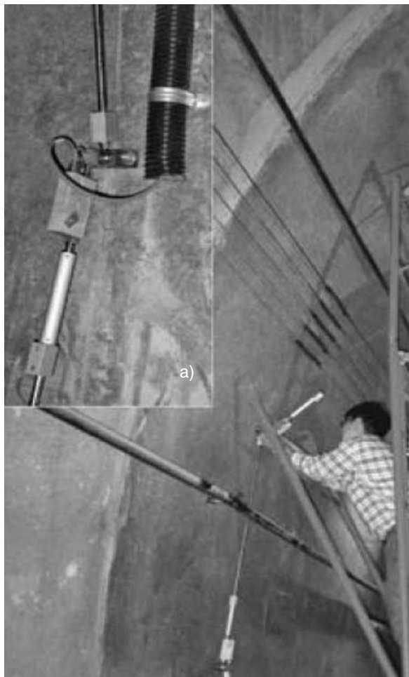
Obr. 2. Tunnel Profile Monitoring System [3]
